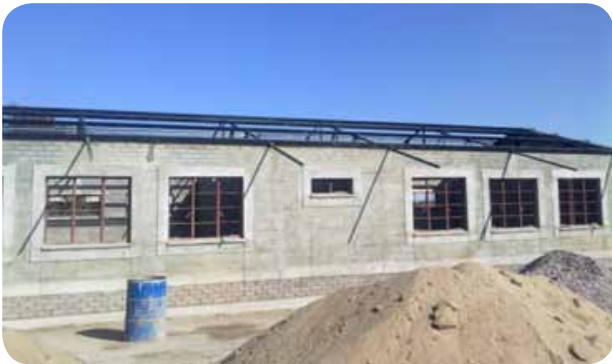
Construction of girls dormitory at Oshela Senior Secondary in Okongo
