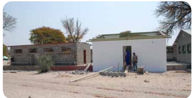
Construction of 2 classrooms in Arandis
