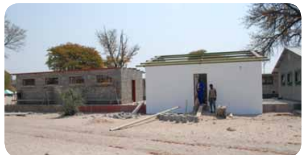
Construction of 2 classrooms in Arandis
