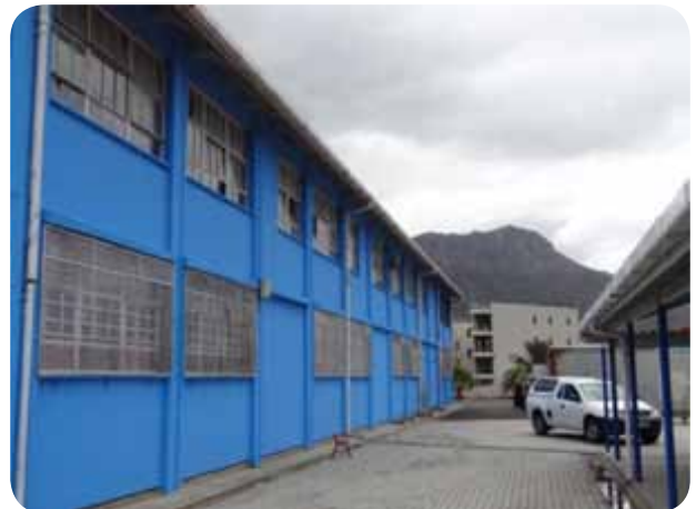
Refurbishment of Sentinel Primary School, Hout Bay
