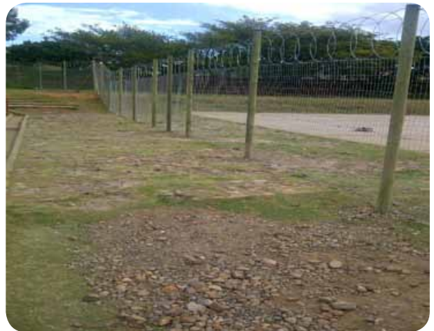
Refurbishment of Papenkuil Primary School, Port Elizabeth
