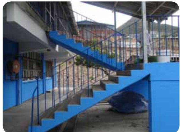
Refurbishment of Sentinel Primary School, Hout Bay
